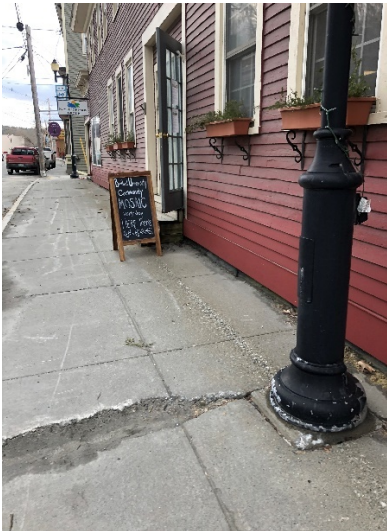
Left: minor cracks in the sidewalk need repair and could be opportunities for integrating art (such as mosaic) into infrastructure. Middle and right: breaks in the sidewalk route and errant snow piles make walking hard on the north/west side of Main Street between the Wall and Bethel Central Market.
