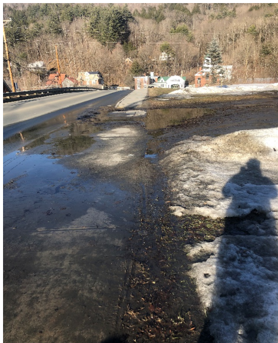
Left: Driveways create breaks in the sidewalk network and collect rainwater and snowmelt on Church Street, leading to hazardous ice and silt buildup.
